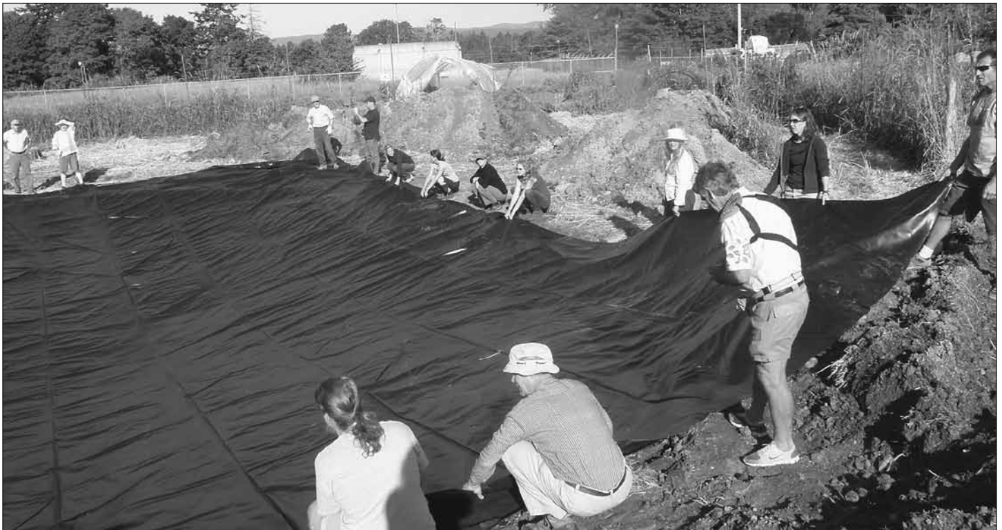
The pond excavation was lined with a layer of geo-textile and the PVC liner placed on top of this layer. A second layer of geo-textile was then laid on top of the PVC liner to further protect it.
