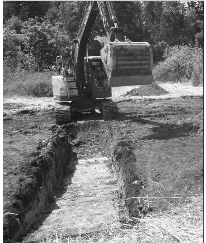
The excavation started by scraping the top soil off to reveal the perimeter of the pond and a trench was dug along the axis to establish depth and slope contours.
